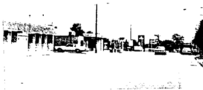
Spread of highway and retail commercial developments
