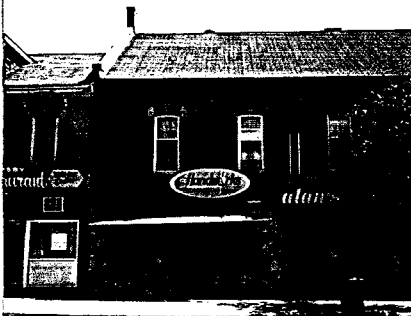
Positive example of a streetscape of buildings utilizing many of their original details and materials.
