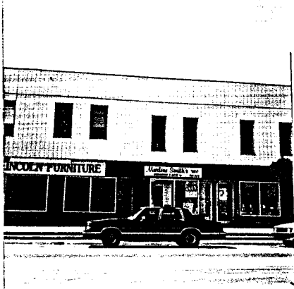
Original facade materials have not been used.
